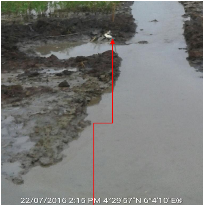
Fig A: Incident Area just before excavation
