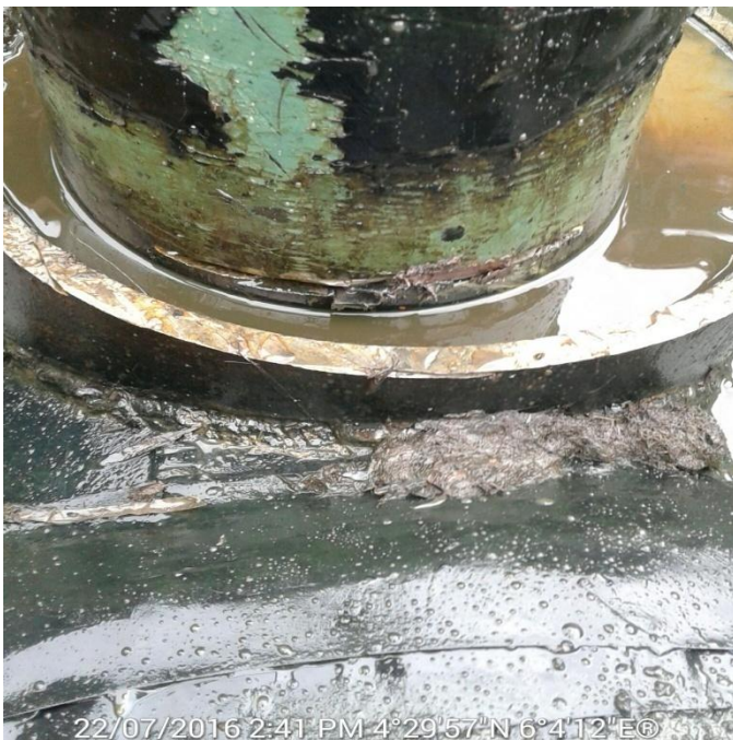
Fig C: Leak point pegged during repair.
