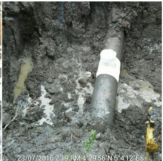
Fig D: Incident Facility after repair.
